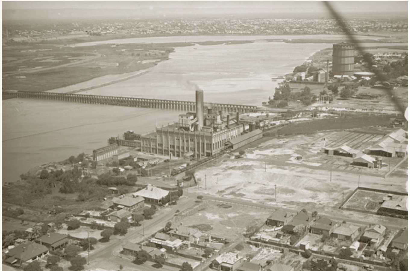
East Perth Power Station c.1930
