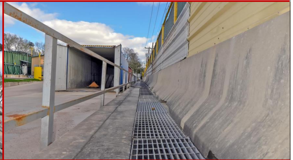
Concrete Barriers with metal Fencing and metal grates for onsite water management
