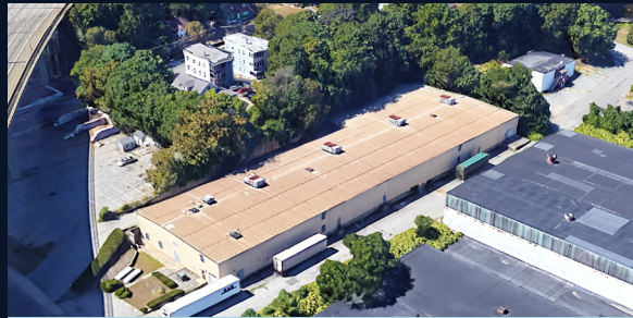
56 Lewis Street, New London, CT ~67,751 SF
