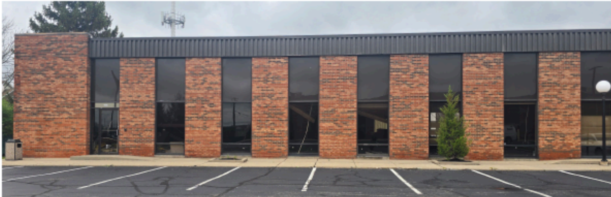
EXISTING CONDITIONS PHOTO
