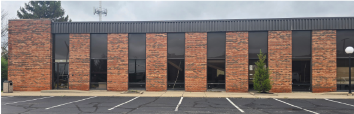
EXISTING CONDITIONS PHOTO
