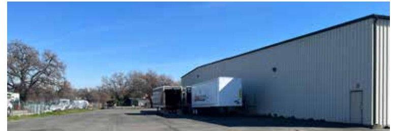
Area C - northwest side
