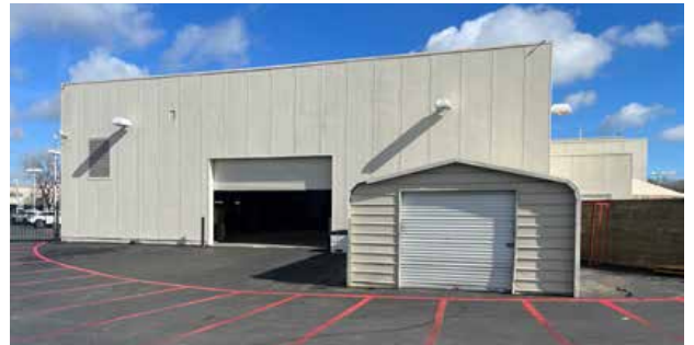
Building south shop entrance
