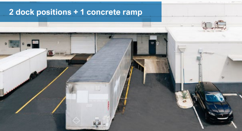
Gated and secured truck court
