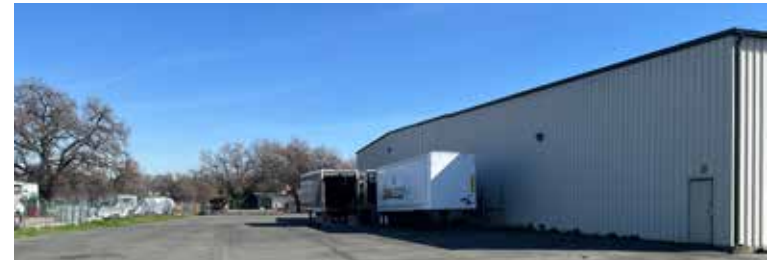
Area C - northwest side
