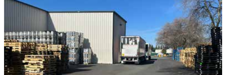
Area B - back view of loading docks
