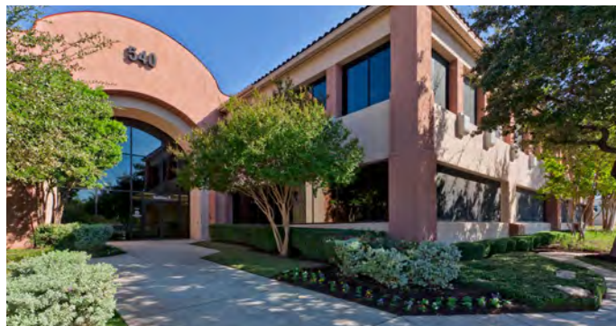
PLAZA II 540 OAK CENTRE DRIVE
