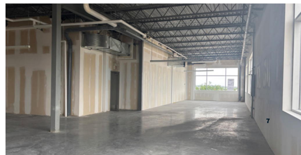
Second floor office opportunities can be combined
