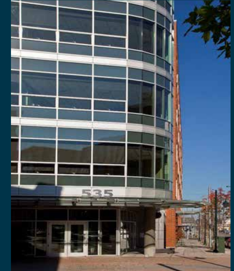
Amazon.com HQ Phase 1B / Interurban Exchange II 115,000 SF / Class A Office Seattle, WA (SLU) Completed 2010; Sold
