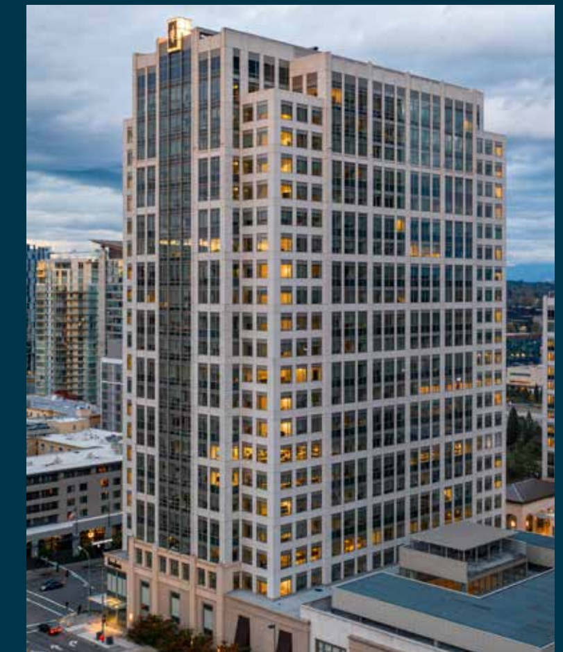
The Bravern Office Commons 749,694 SF / Class A Office Bellevue, WA (CBD) Completed 2009; Sold
