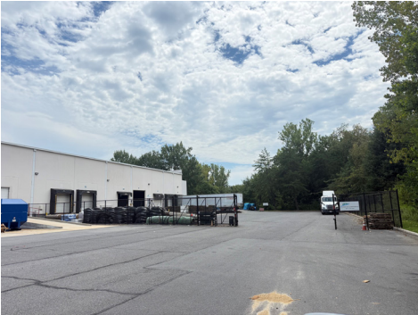
Fenced Truck Court
