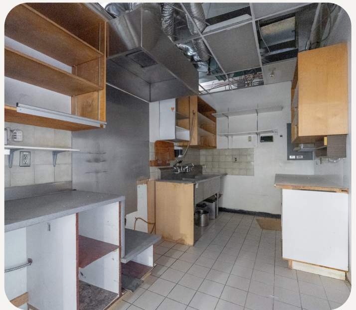
Unit 202 ( kitchen interior )
