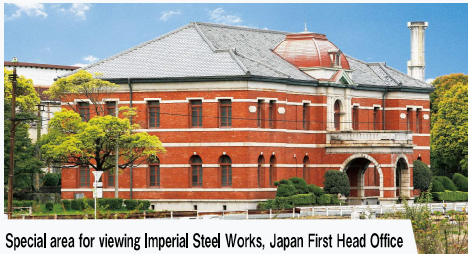
Special area for viewing Imperial Steel Works, Japan First Head Office
