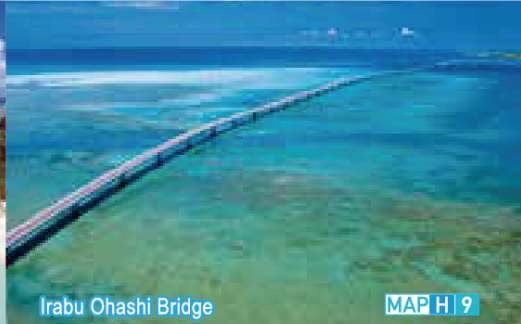
Irabu Ohashi Bridge
