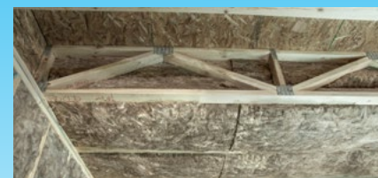
Inner-Safe batt insulation installed in Open Web interstitial space.
