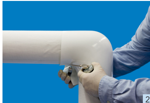
Using a standard applicator gun or squeeze bottle, apply a bead of Proto's solvent weld adhesive between the overlap of the PVC fitting cover.
