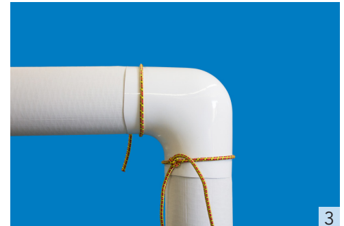
Press the fitting cover into place and temporarily secure using a tourniquet, elastic cord or PVC tape.
