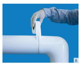
For an attractive finish, apply Proto's PVC tape around the circumference of the butt joints.
