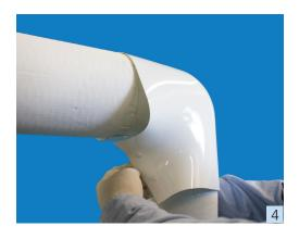
Insert stainless steel serrated tacks (2+ tacks per fitting) approximately ¼" (6mm) from one of the lap edges of the fitting cover. For large or specialty fitting covers, use additional tacks to obtain a smooth, uniform fit. To assist with tack installation, form a small hole on one side of the fitting cover (using an awl or hole punch).
