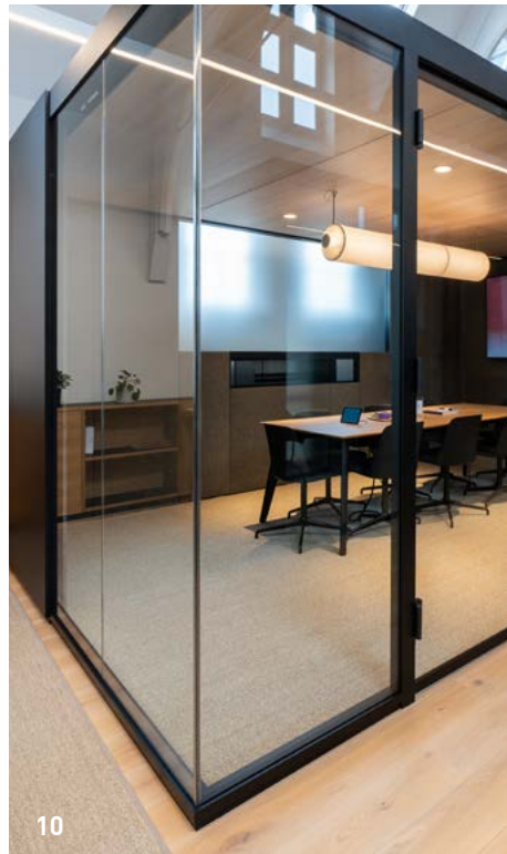
10 | Perfectly formed Glass corners on butt joint with transparent corner profile
