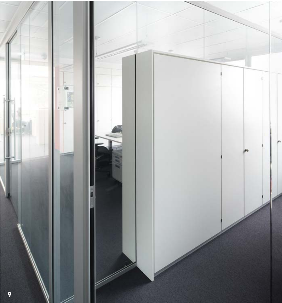
8 | Perfect Ceiling-high doorframe and butt-jointed glass corner. 9 | Segmented The storage wall is glazed.
