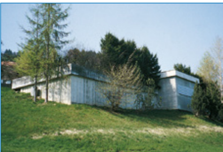
Reservoir Aesch, Stufenpumpwerk, 1976
