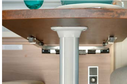
Extruded, anodized aluminum to be strong and lightweight
