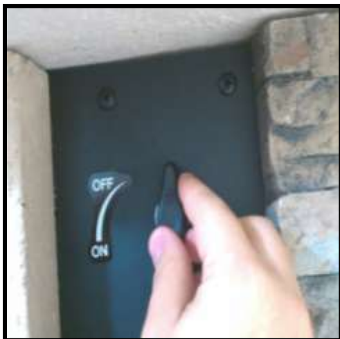
Step 2. Shut off gas valve at appliance.
