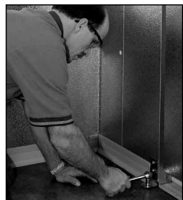
Attach slam brace with fastener provided
