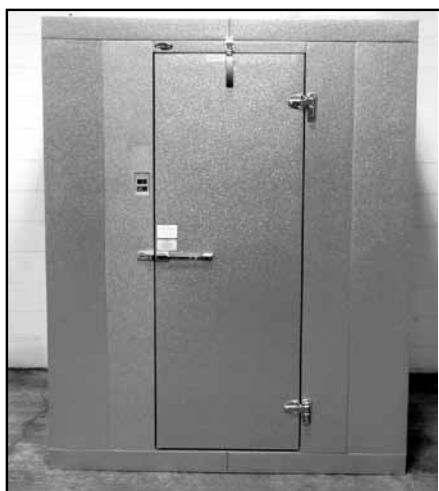
Completed Walk-in with floor
