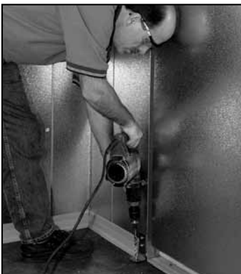
The recommended hole size for PARABOLT ANCHOR is 3/8" X 2-1/4"
