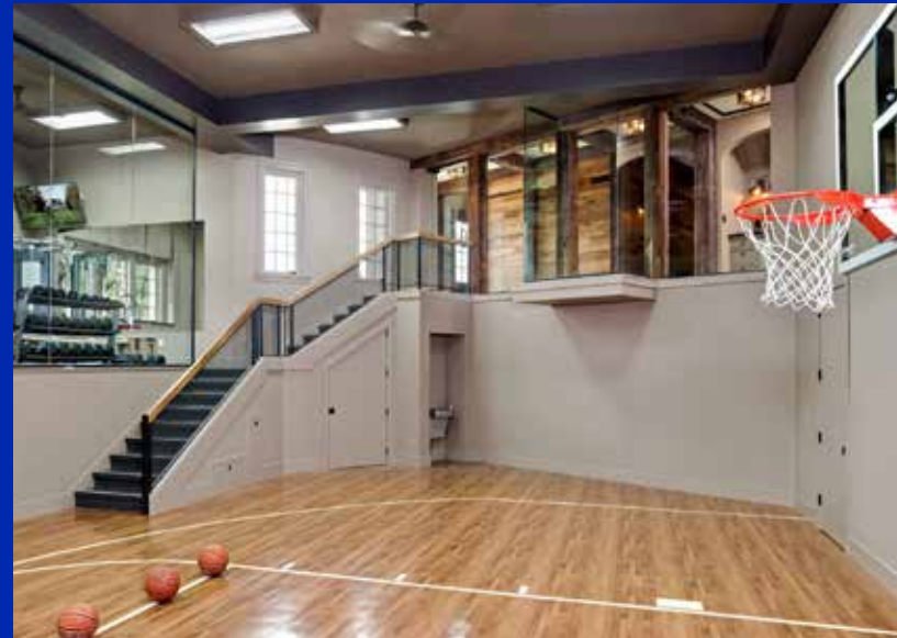
NEW GLASS HANDRAIL OVERLOOKING BASKETBALL COURT BELOW
