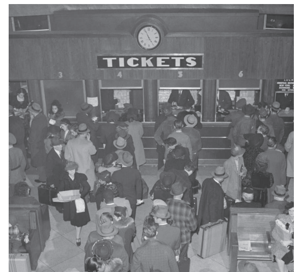
BUS TERMINAL LOBBY 1100 NEW YORK AVE JAN 1941
