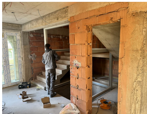
The elevator shaft being installed.
