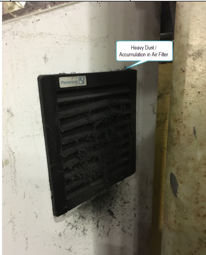
Figure 5:2 - Mill #2 Rea-JET Cabinet Filter
