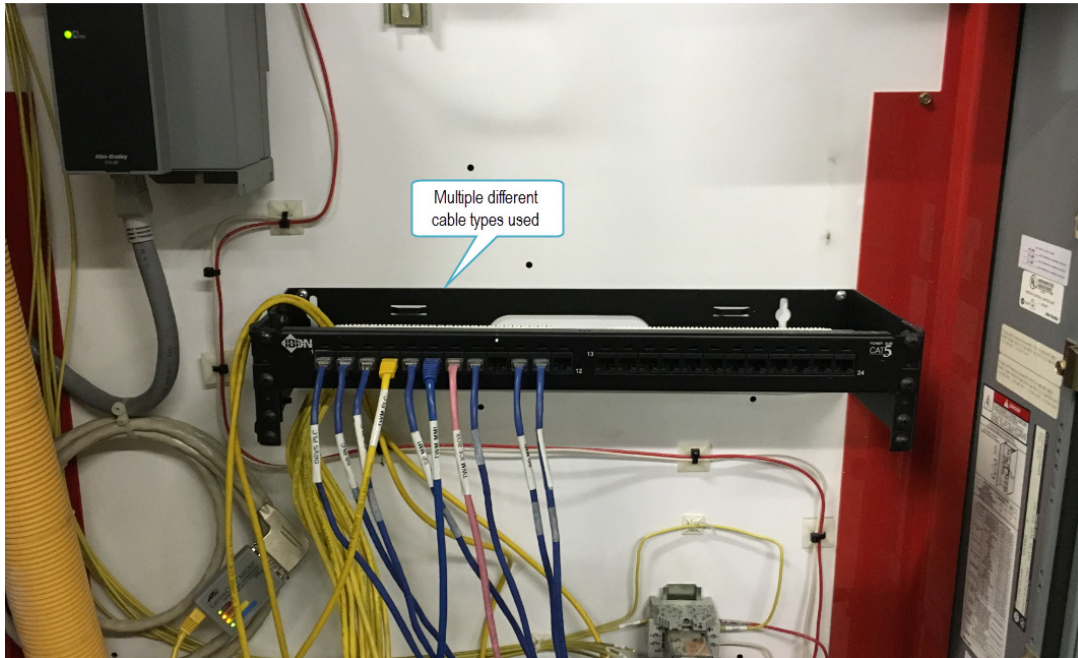
Figure 5:4 - Mill #2 TWM Cabling
