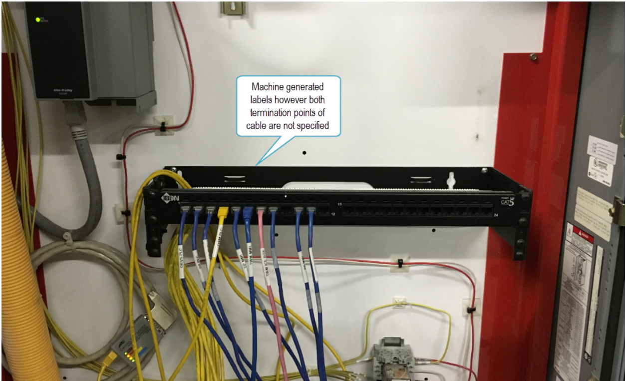
Figure 5:17 - Mill #2 TWM Panel Cable Labeling
