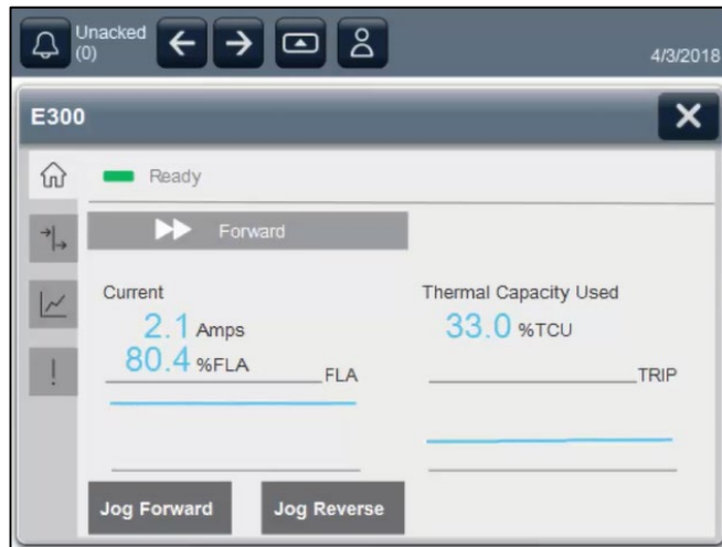
Device Status & Maintenance Control
