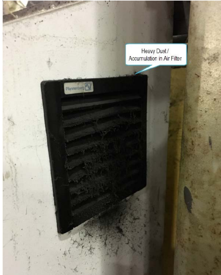
Figure 4:3 - Mill #2 Rea JET Cabinet Filter
