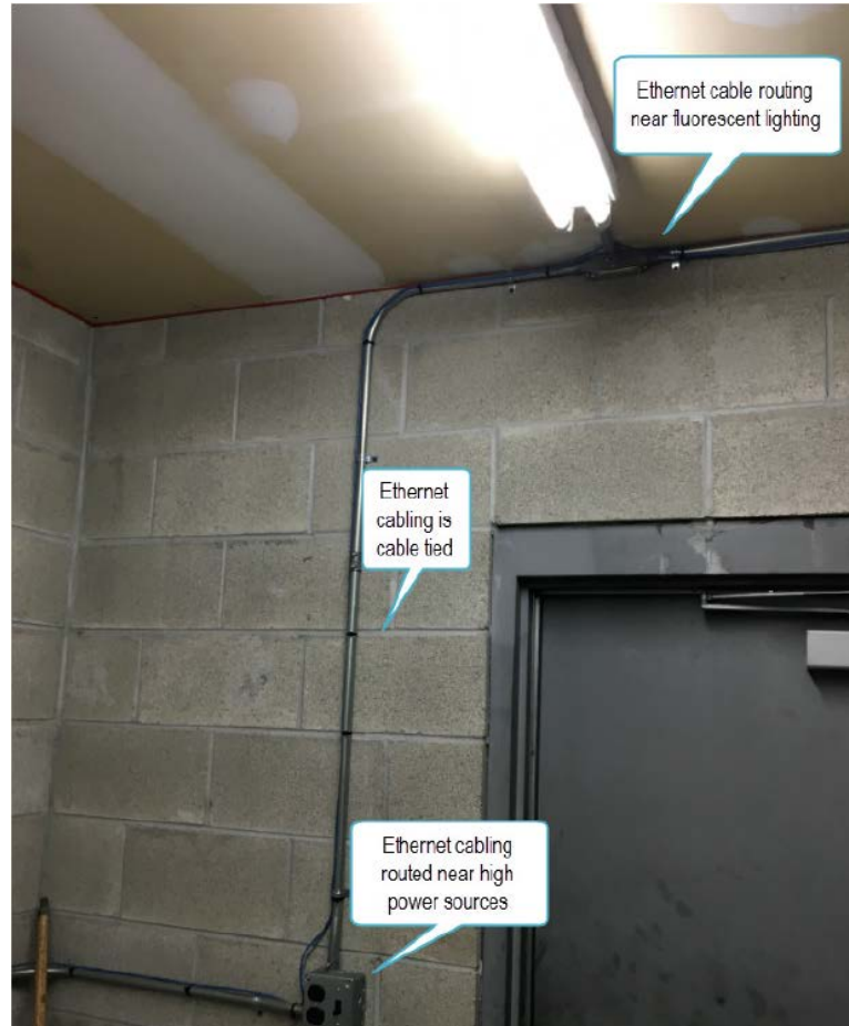
Figure 4:12 - Slitter #4 Drives Room Cable Routing
