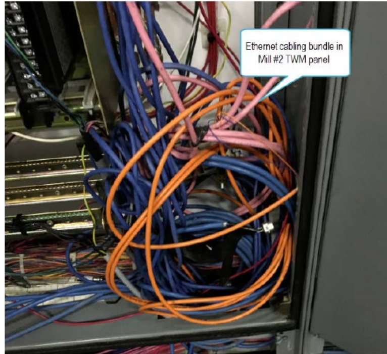
Figure 4:6 - Mill #2 TWM Panel Cable Routing
