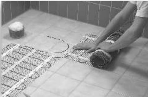
When approaching obstacles (toilets, cabinets, etc.), carefully remove some of the red heating cable from the mat and lead the cable around the obstacle. In some cases pieces of the grey mesh will be cut away entirely. Remember to never cut the red cable. Use hot melt glue or a thin strip of tape to secure the loose cable to the floor.
