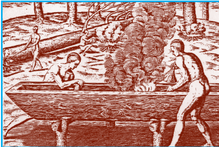
Shaping of a canoe by controlled burning.
