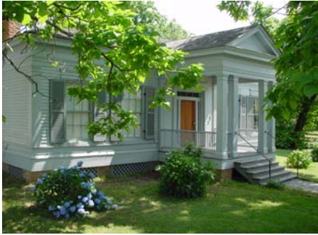
The Augustus Crouch House, built in 1856, showcases exhibits on historic tools and construction techniques.
