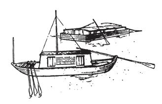
Several methods were used to gather shells, including simple hand collection in which mussels were harvested individually. Specially equipped boats called "shelling rigs" allowed collectors to harvest many shells at once from known mussel beds. Shelling usually provided a supplementary income.
