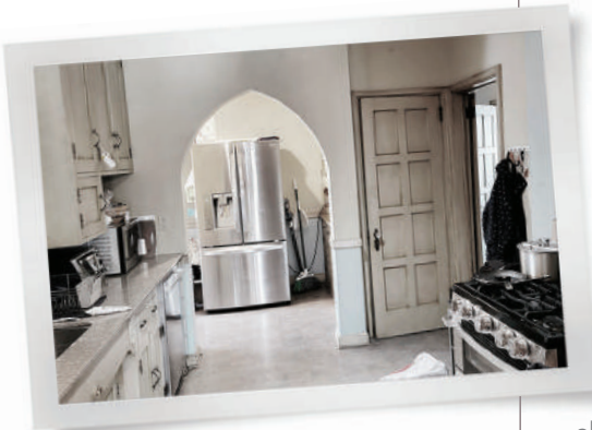
A 1980's remodel had not served this house or kitchen well.
