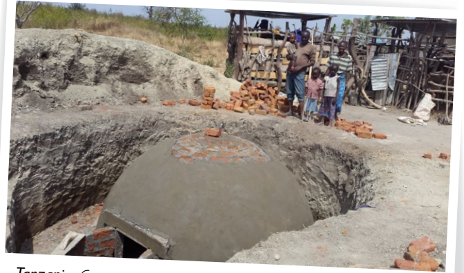
Tanzania: Constructing one of several underground tanks that make up the biogas system. World Vision
