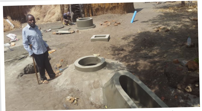
Tanzania: Once the tanks are buried, only the tops are visible. The tall pipe in the background is the first tank where water is mixed with manure. The square top is the tank where the gas pipe connects, and the front tank is for the waste. World Vision
