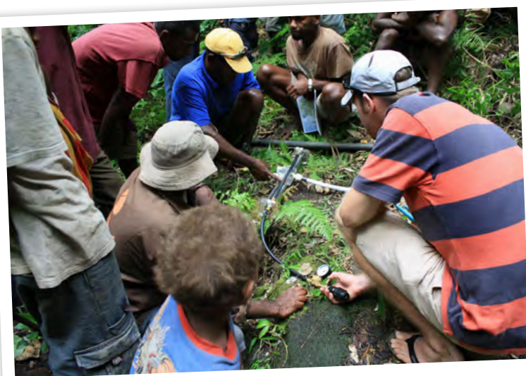
Vanuatu: Community members work with a World Vision engineer to pipe water from the source to community access points. Elizabeth Brown
