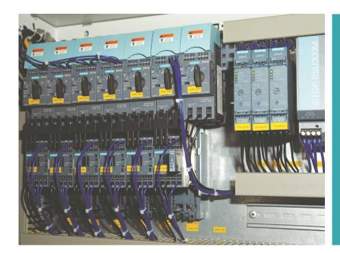
The Siemens 3RV29 infeed system is much less labor intensive.
