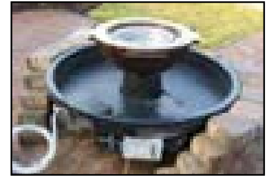
360 Feature being finished with paver stone Includes Basin, 26" Copper Water Bowl, and Electronic Ignition Fire Pit (13SSEI).
