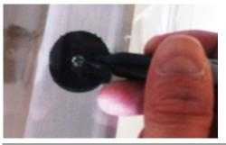
**4.** Using the provided self tapping screws, attach all the hardware for your cover. Be certain to attach the Dual-Lock™ in the center of the well wall.
