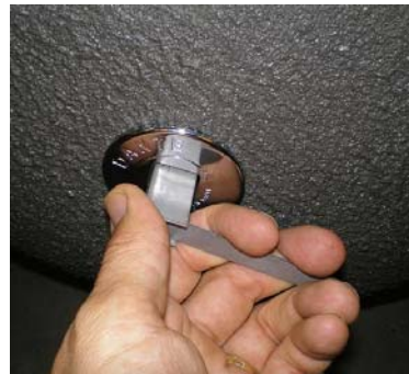
Tighten Key Way with Tool.
