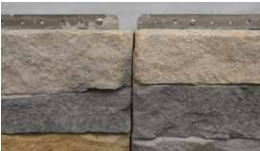
Poor choice of mating panels. Panel stone sizes are too similar from panel-to-panel.
