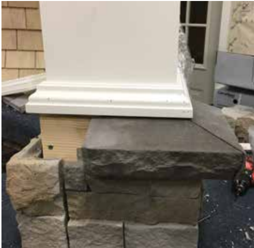
STONEfaçade sill piece or Restoration Millwork trim pieces to cover the top of STONEfaçade panels.
