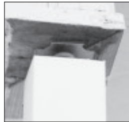
8. Position top of post directly under the top fastening plate.
