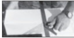
3. If using handrail, check local building codes for minimum rail height. Decide how much is to be trimmed from each end of PermaPost. Top and bottom mounting plates are 1/8" thick. Mark post 1/4" shorter than total opening.
