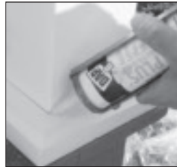
12. Slide skirt into position and caulk seam.
