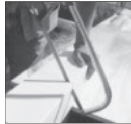
4. Using a hacksaw, trim the post at top and bottom.
