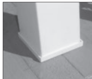
6. Position bottom of post over bottom fastening plate.
