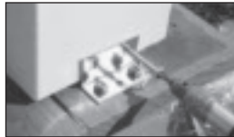
11. OPTIONAL FASTENING METHOD SOLD SEPARATELY. Follow directions above except slide skirt over post prior to positioning. Attach corner irons to post and floor with supplied screws.
