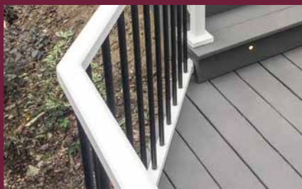
Special Welded Corners
