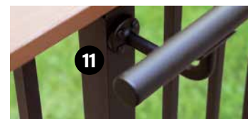
Extended Wall Mount Detail
