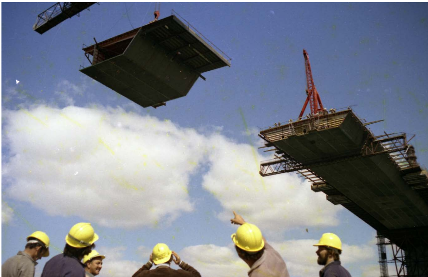
The West Gate Bridge under construction.
