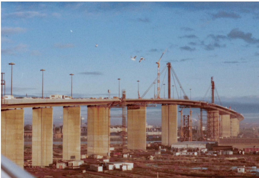
The West Gate Bridge was completed in 1978.
