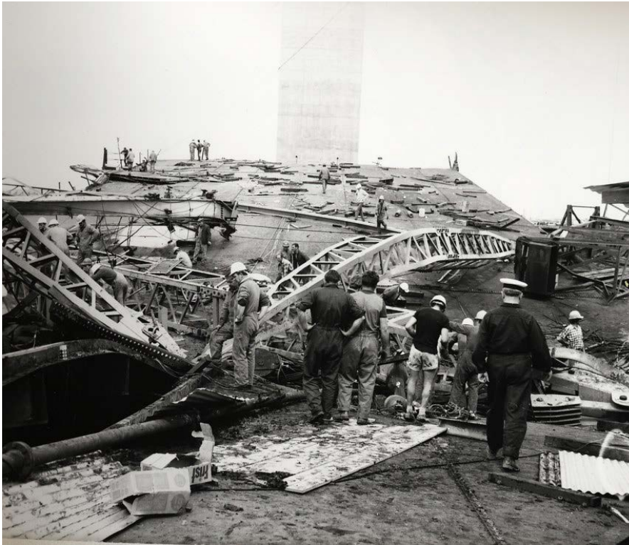
Wreckage of the collapsed bridge Photo: Public Records Office of Victoria
