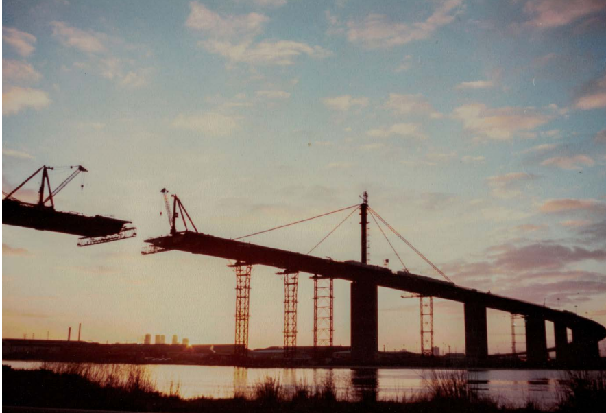
The nearly-completed West Gate Bridge.
