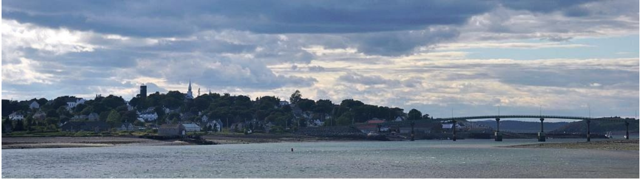
Figure (32) FDR Memorial Bridge
