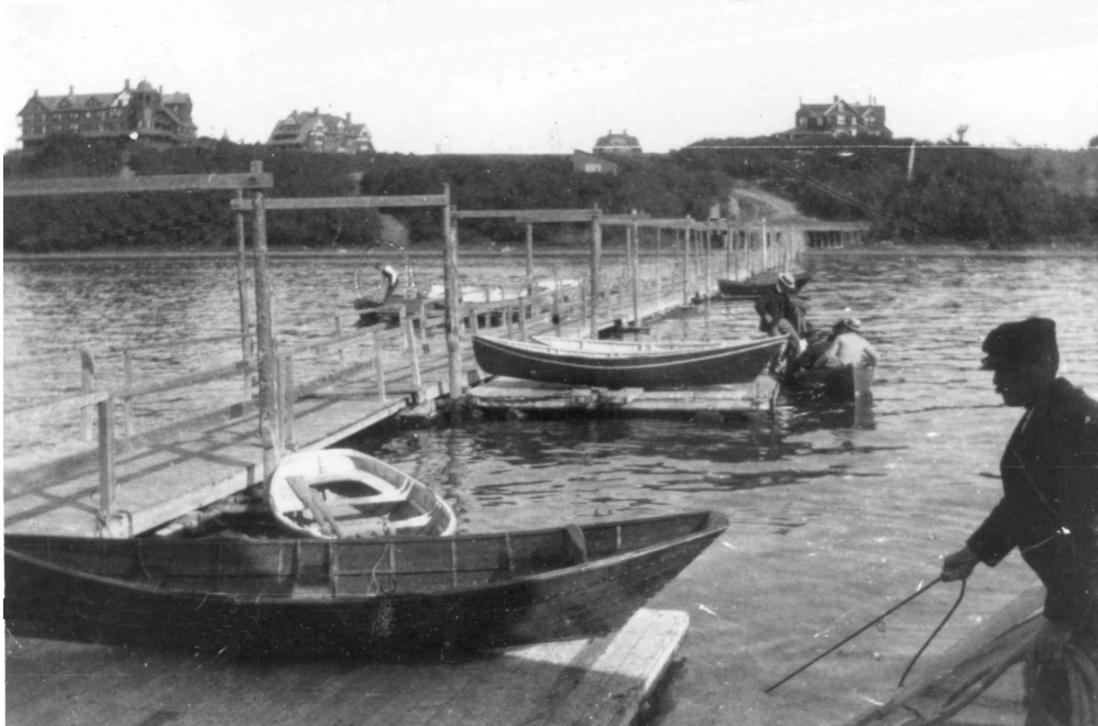
Figure (3) 1904, The Floating Docks Hotels and a cottage can be seen in the background.
