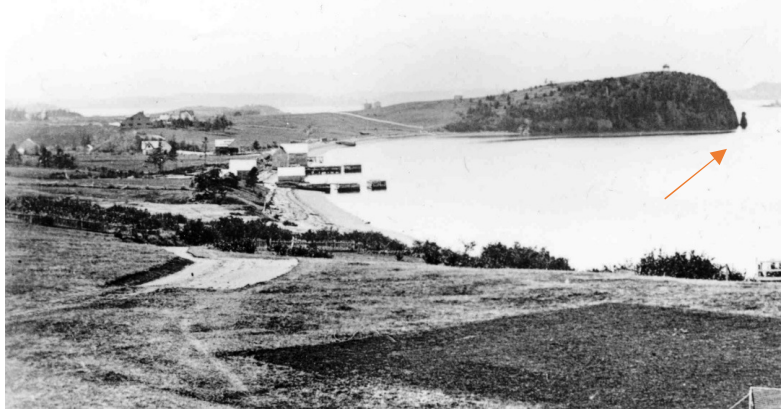
Figure (1) 1882, Friar’s Bay : View Of Hotels And Cottage Construction
