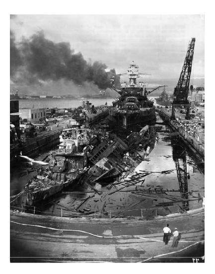
The destroyers *Downes* (left) and *Cassin* (right) in dry dock; the *Pennsylvania* [the flagship of the Pacific Fleet] is in the rear. The machinery and fittings of the *Cassin* and *Downes* were salvaged and used in new hulls. The *Pennsylvania* suffered only minor damage.
