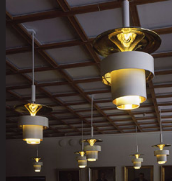
Ceiling fitting National Pensions Institute, head offices
