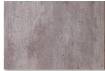
2204-K00 S Cracked Cement
