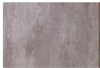
2204-K00 S Cracked Cement
